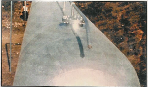
Application of zinc tape on Fuel Tanks.
